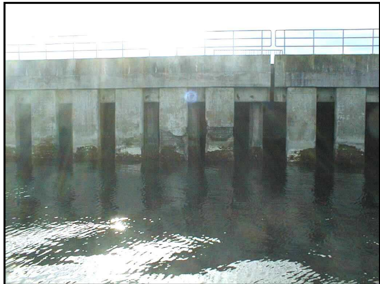
Figure 2-39. Pier B wave attenuation baffles.
